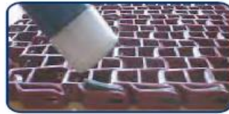
After rod is positioned, place plug and drive it in position with a hammer.
